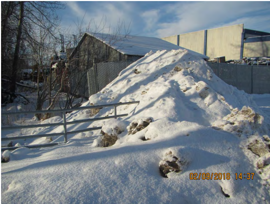
S. Fork Little Campbell Creek at Petersburg--snow from the parking lot has been pushed up to the edge of the creek which is illegal. When it melts, there will be all sorts of trash and pollutants, e.g vehicle drips and ice melt chemicals, entering the creek.
