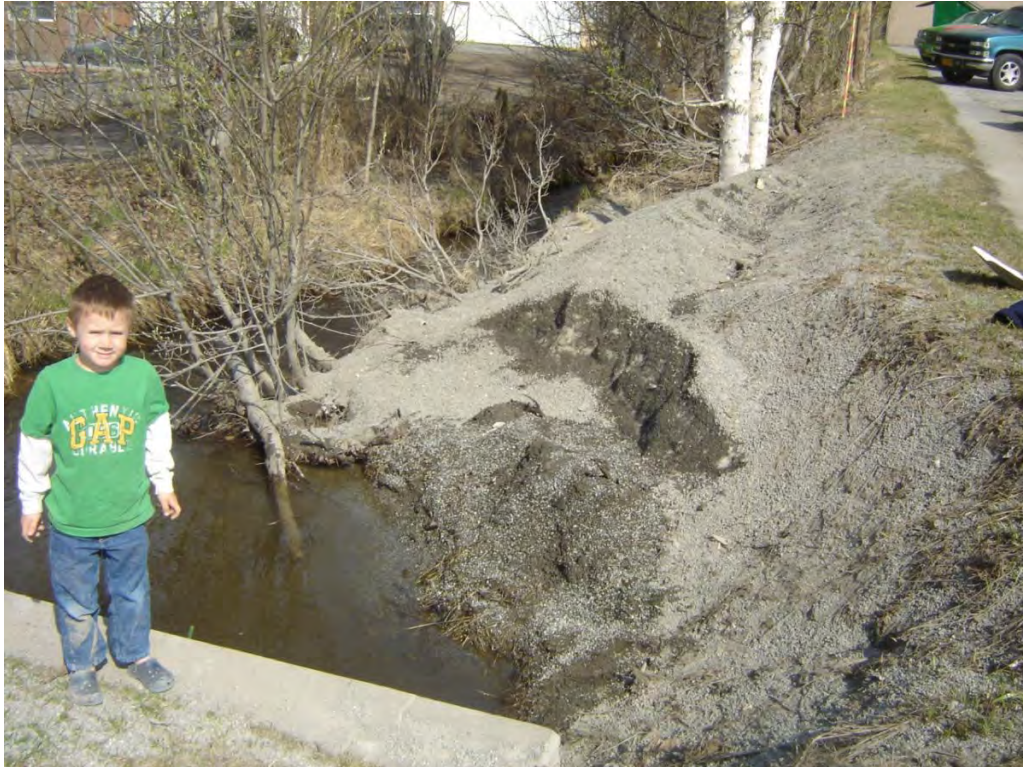
S. Fork Little Campbell Creek at 76th and Old Seward--snow disposal from the parking lot was at the edge of the creek, which, when melted, left piles of road sand and gravel tumbling into the creek.
